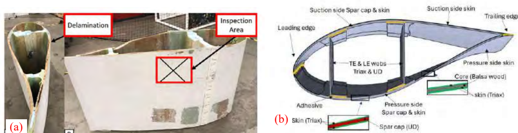
Fig. 1. (a) Delamination in WTB [5]; (b) Cross-sectional view of the WTB [6].
